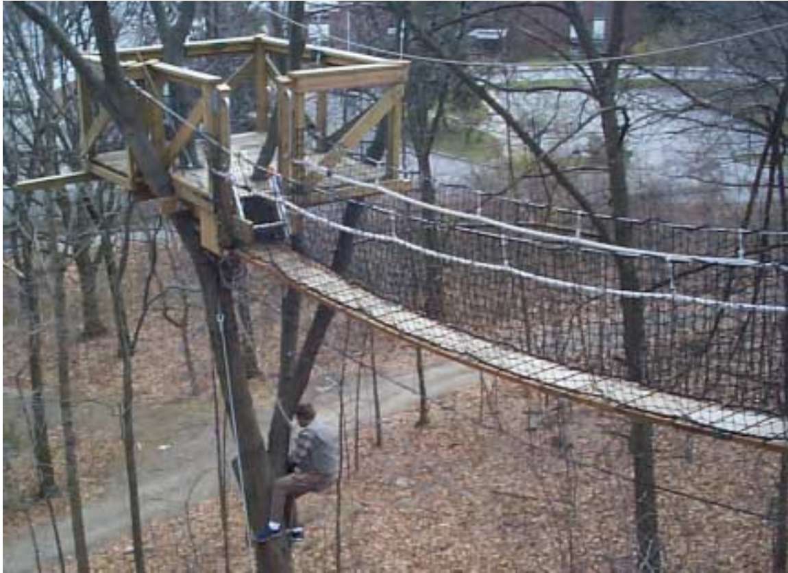
Figure 1 Photograph of walkway during construction at The EcoTarium, Worcester, Massachusetts.
